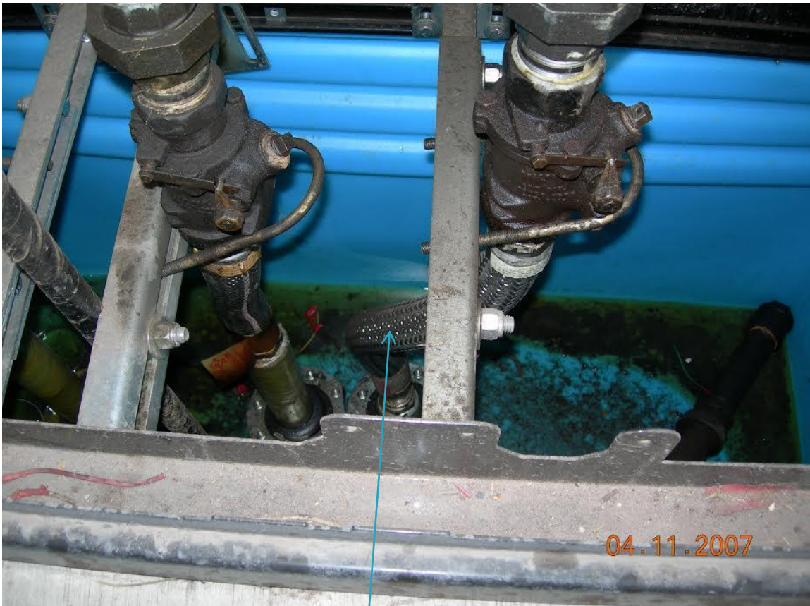
Flex Connector at a dispenser
