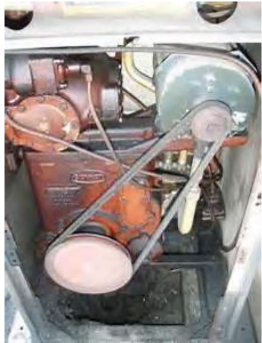
pump under dispenser – suction
